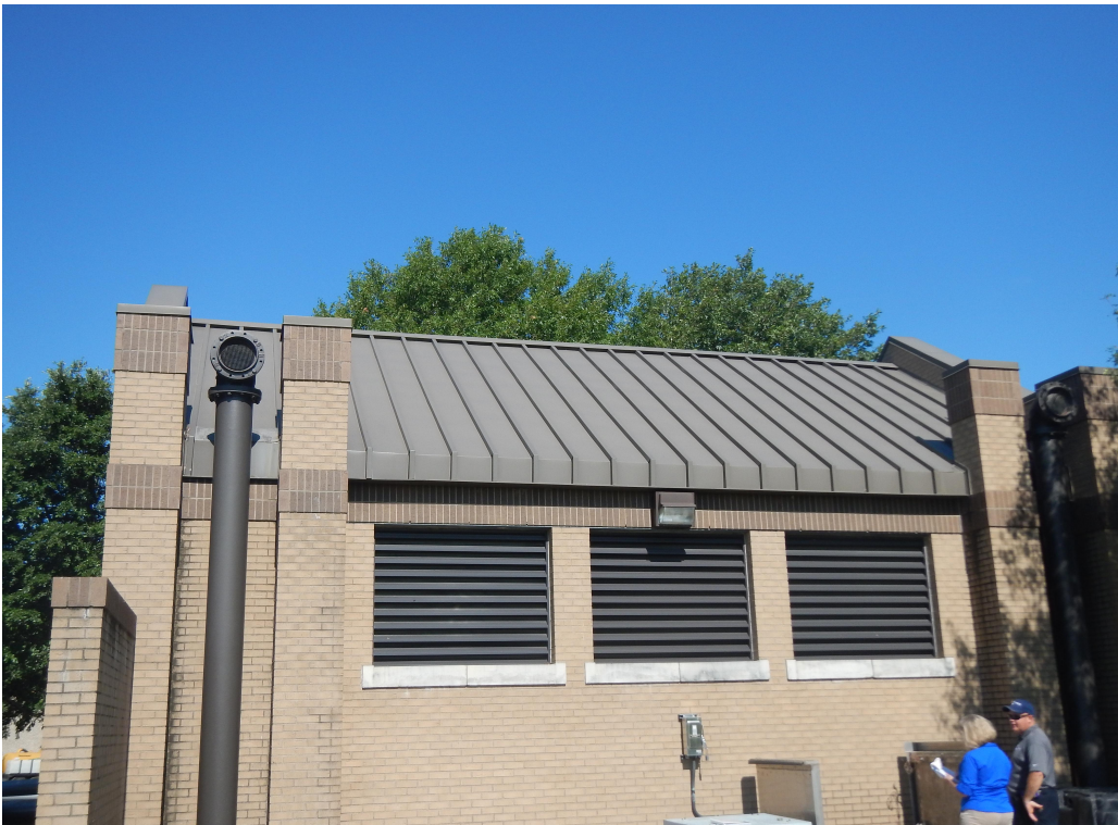
Control Room Roof - Exterior East Side View
