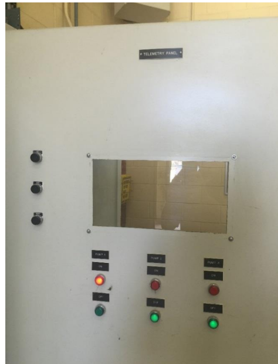
Figure 2-2: SCADA/Telemetry Panel
