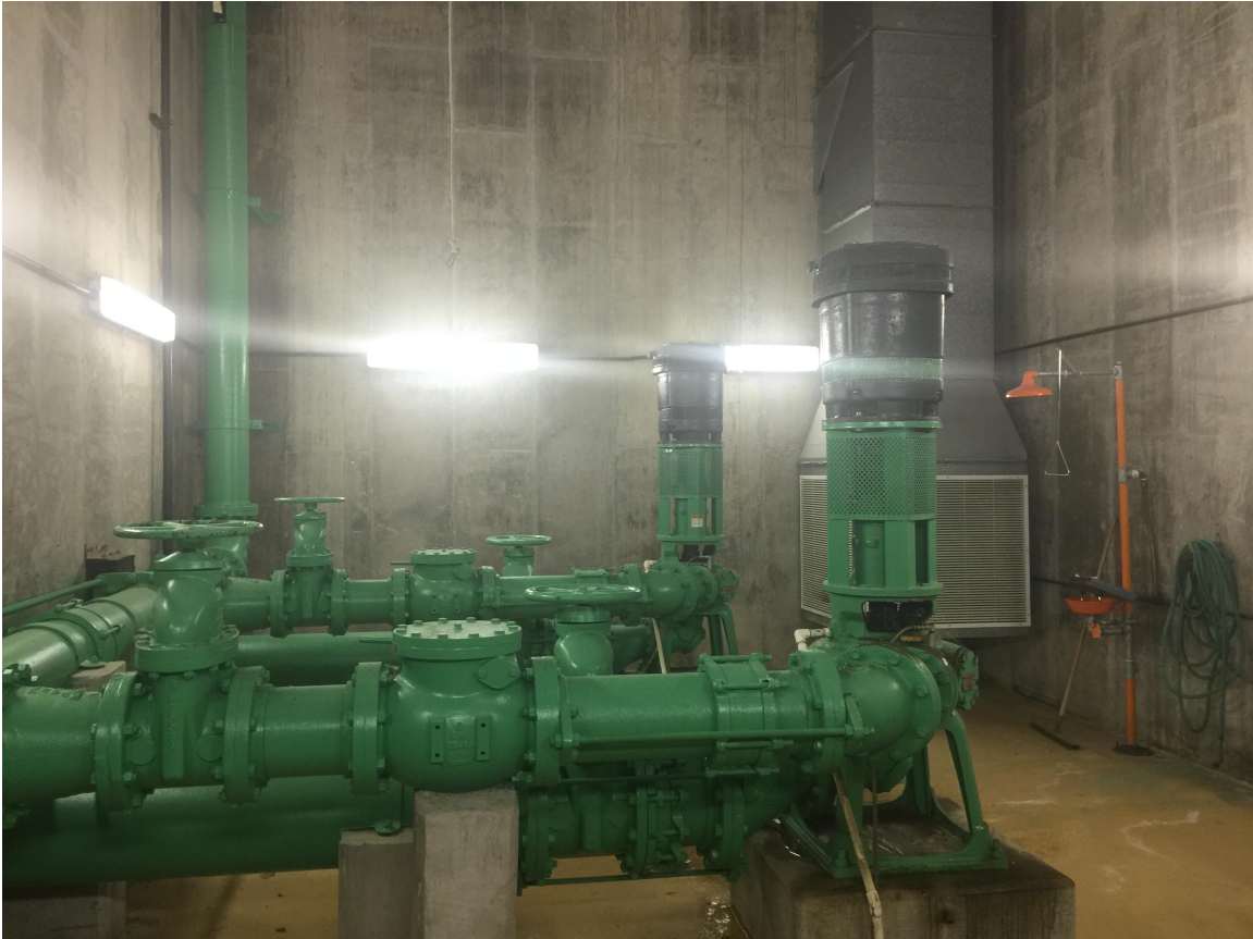
Pump Room Structure - Looking South
