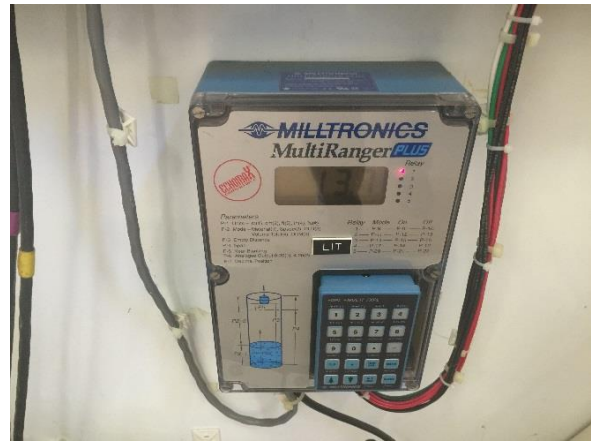
Figure 2-4: Milltronics Multiranger
