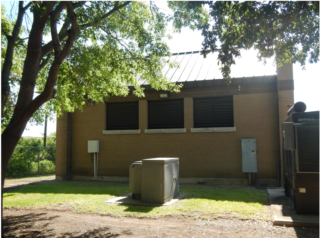
Control Room Structure - West Elevation
