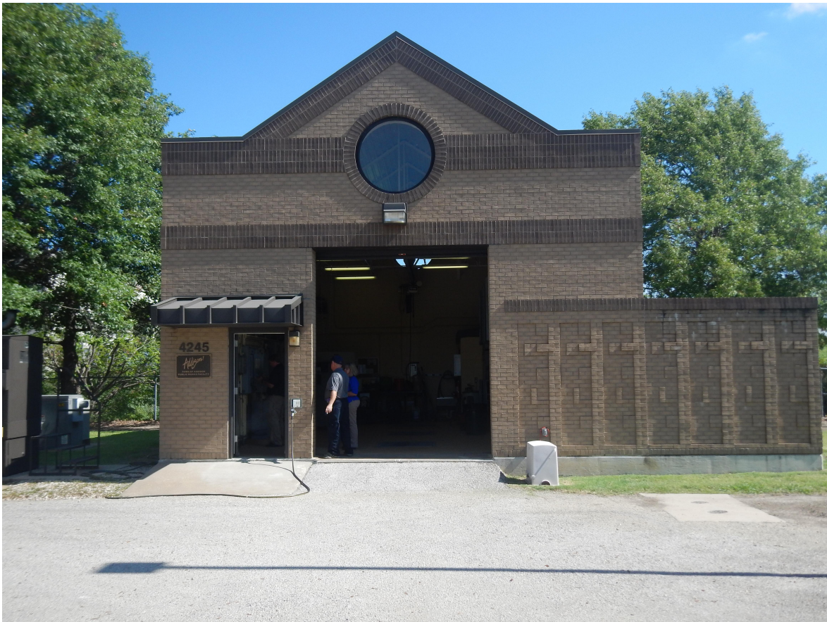
Control Room Structure - South Elevation
