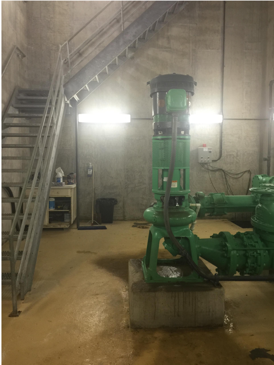
Pump Room Structure - Looking North
