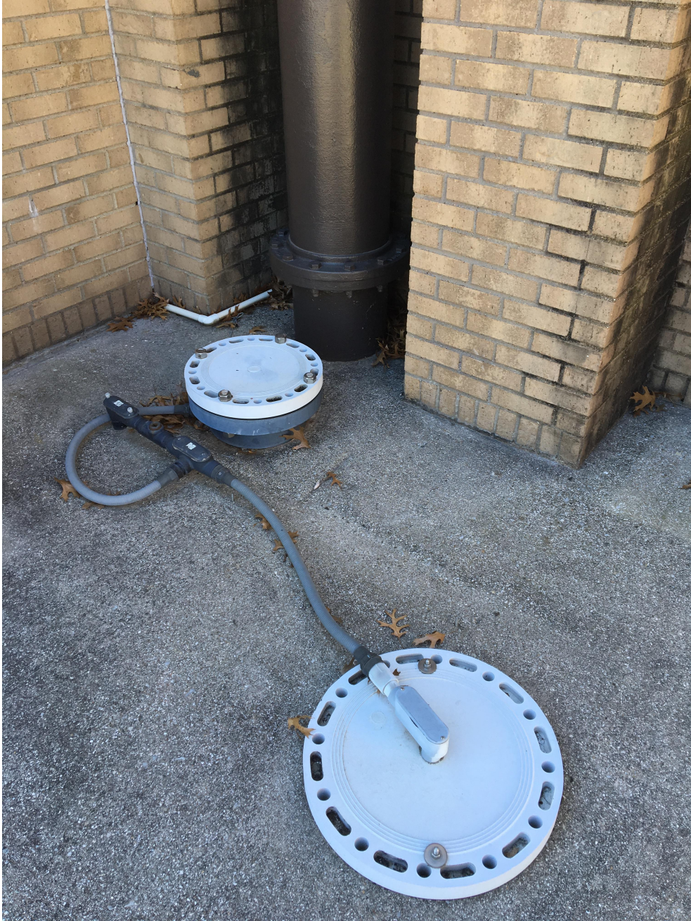
Ultrasonic Level Sensor
