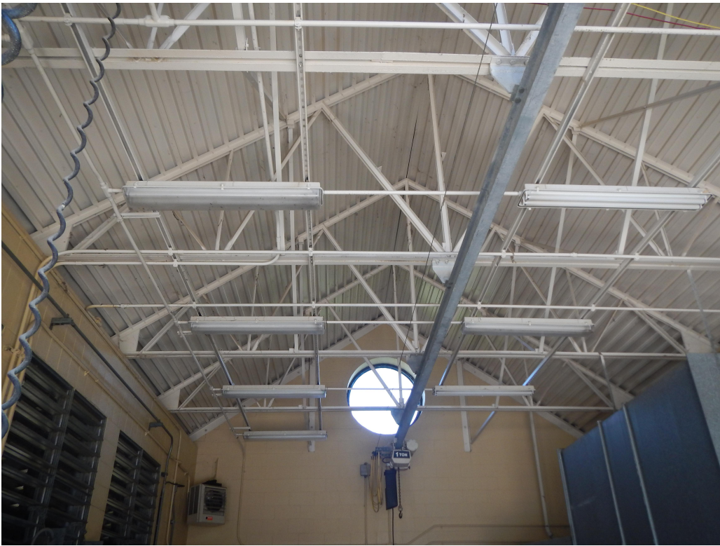
Control Room Roof - Interior View
