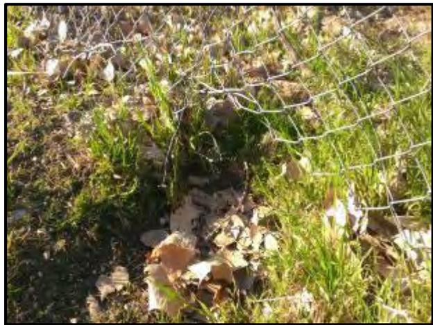
Gates shall remain closed and locked when not in use. Open or unsupervised gates void the integrity of the security perimeter fence and should remain closed when not in use. Gaps to allow for ground clearance and attachment to posts should be no greater than 3 inches. Weekly fenceline checks will continue to identify and fill/repair any gaps.
